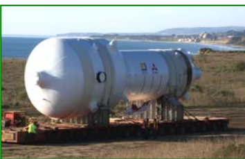
San Onofre's first new steam generator moves toward the plant
