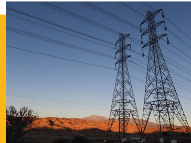
To minimize environmental impact in the West of Devers Project, SCE removed and replaced conductors and supporting structures within a corridor containing existing transmission lines. The corridor spans several communities within Riverside and San Bernardino counties, as well as the reservation trust land of the Morongo Band of Mission Indians.
