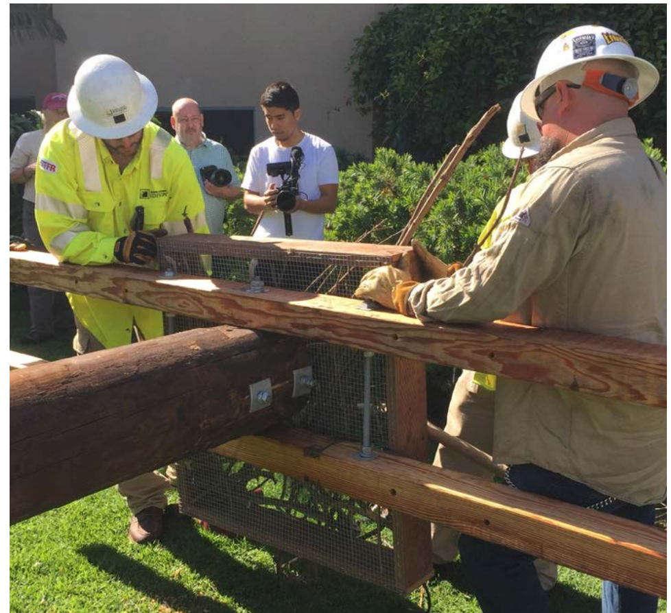
▶ An SCE crew attaches a wood and wire osprey nesting platform to a power pole at Loyola Marymount University.
