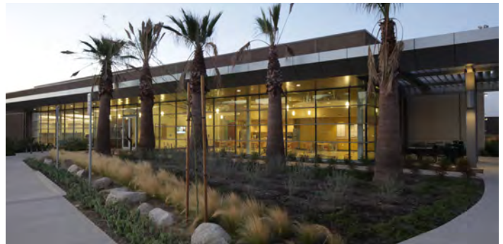
Alhambra Data Center, the newest LEED-certified facility.
