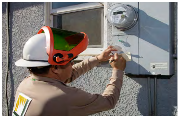
Field Service Representative performing work on a smart meter.
